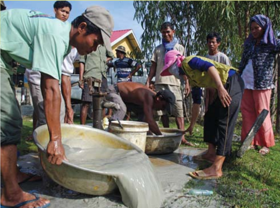
Washing the media prior to filling the filter.
