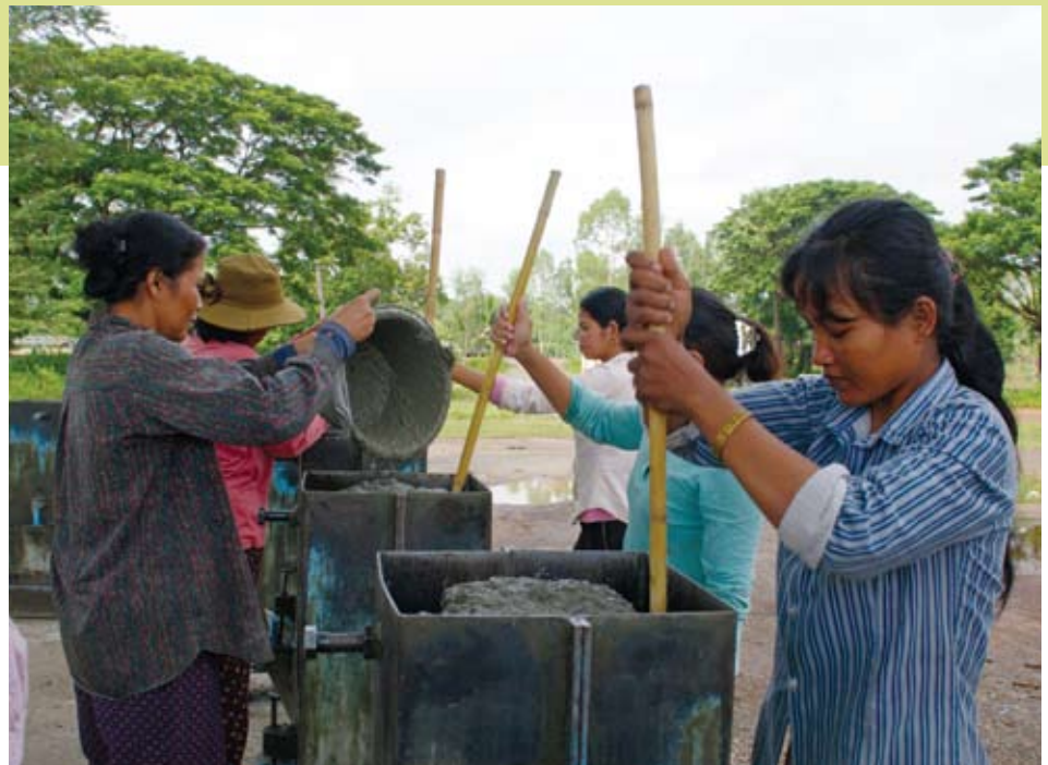
Families play a role in producing their own filter, here filling the mould with concrete.
