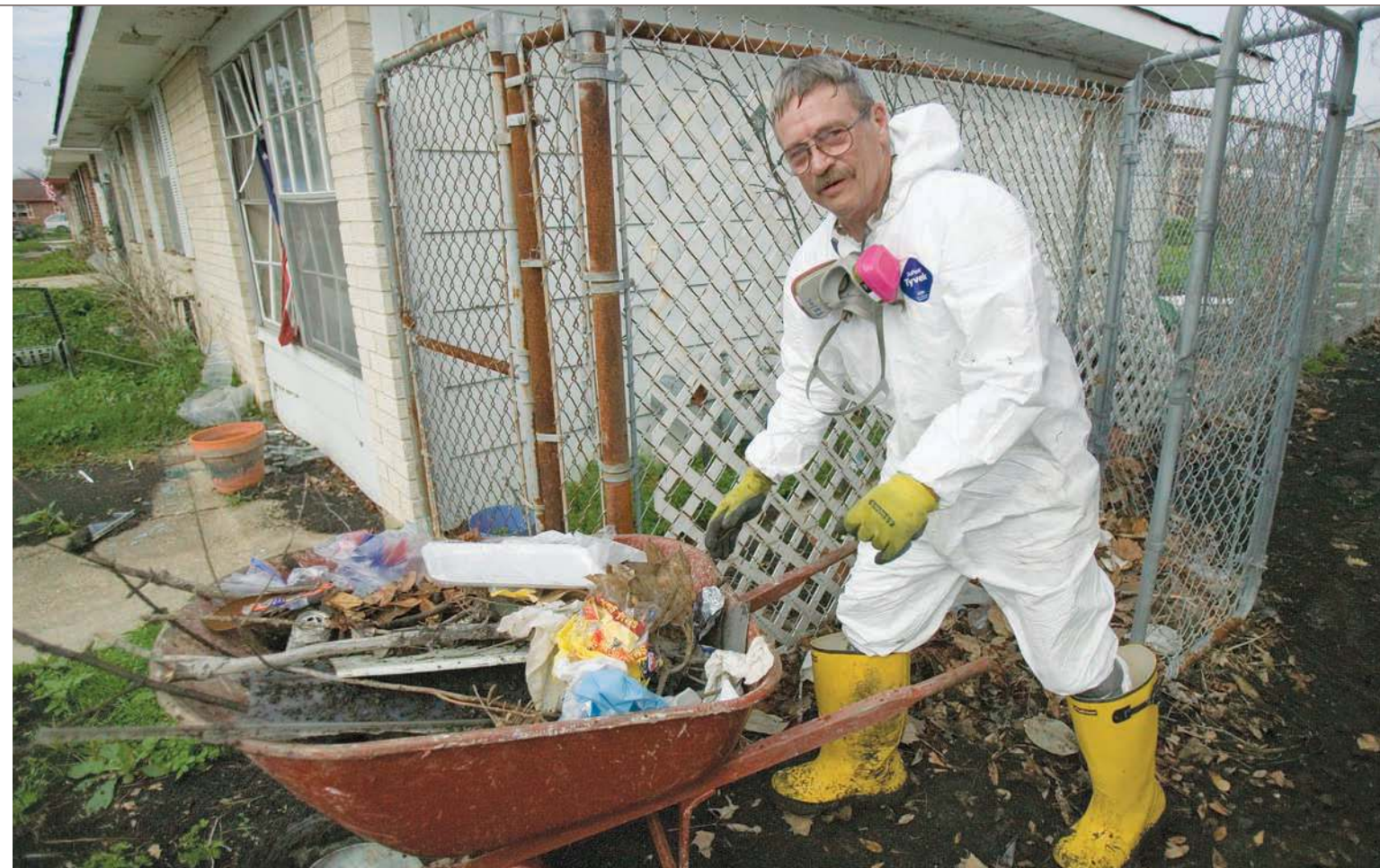
MESSY WORK: Volunteers with our Disaster Relief Unit in the New Orleans area removed mud and muck from more than 1,140 homes, getting them ready for rebuilding.
