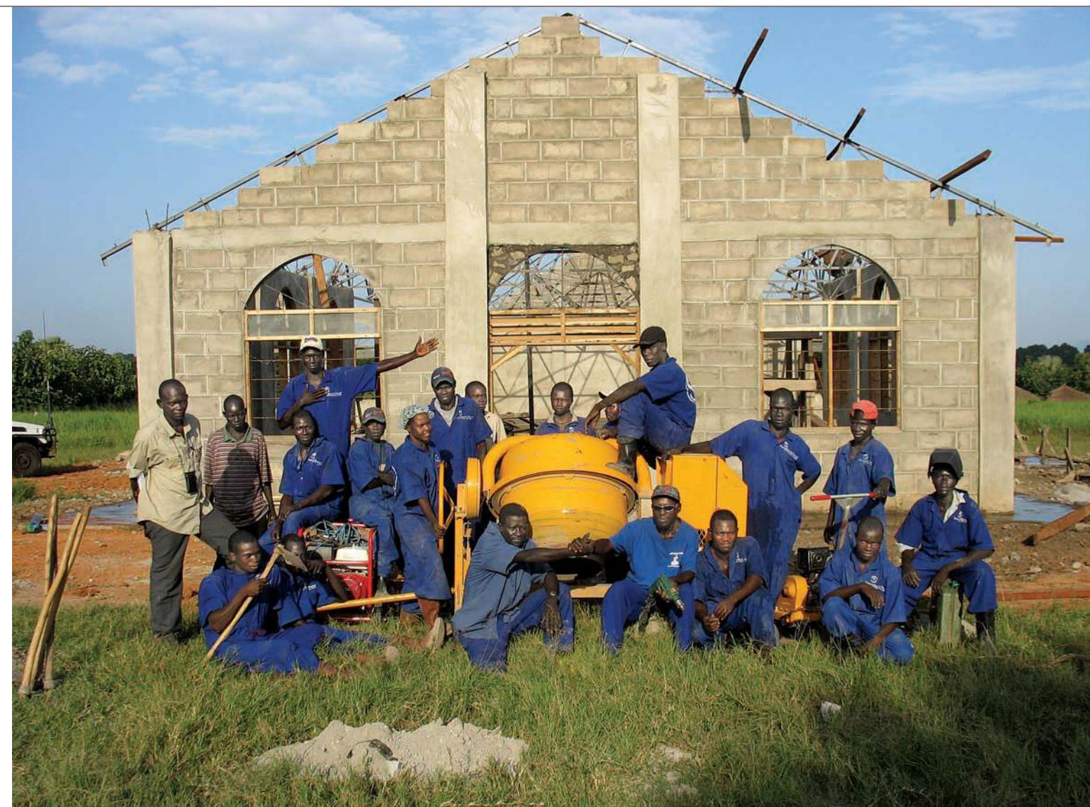
REBUILDING HOPE: Working hand-in-hand with local believers, Samaritan's Purse rebuilt 11 churches in South Sudan, including this one in Lizira.
