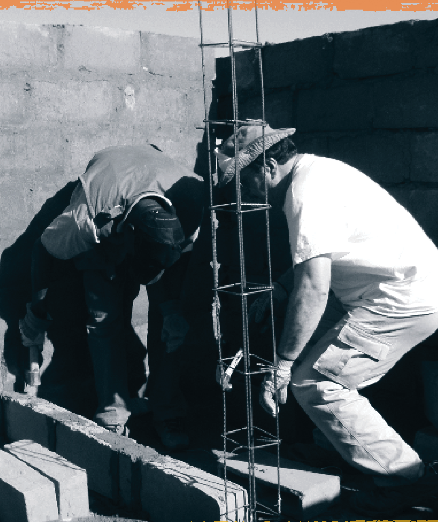
WORKING TOGETHER: From constructing a latrine in Niger to removing water-logged debris from basements in Chilliwack, BC, hundreds of Canadian volunteers worked alongside their neighbors bringing help and hope.
