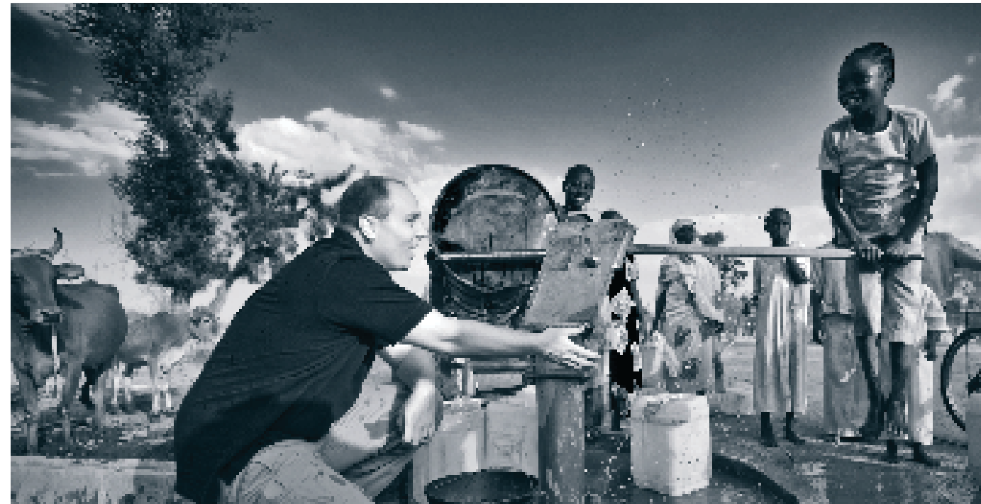
PRIMING THE PUMP: We installed or rehabilitated wells at dozens of locations in Sudan, including this pump near a Bible school built by Samaritan's Purse to train pastors and evangelists in the Nuba Mountains.
